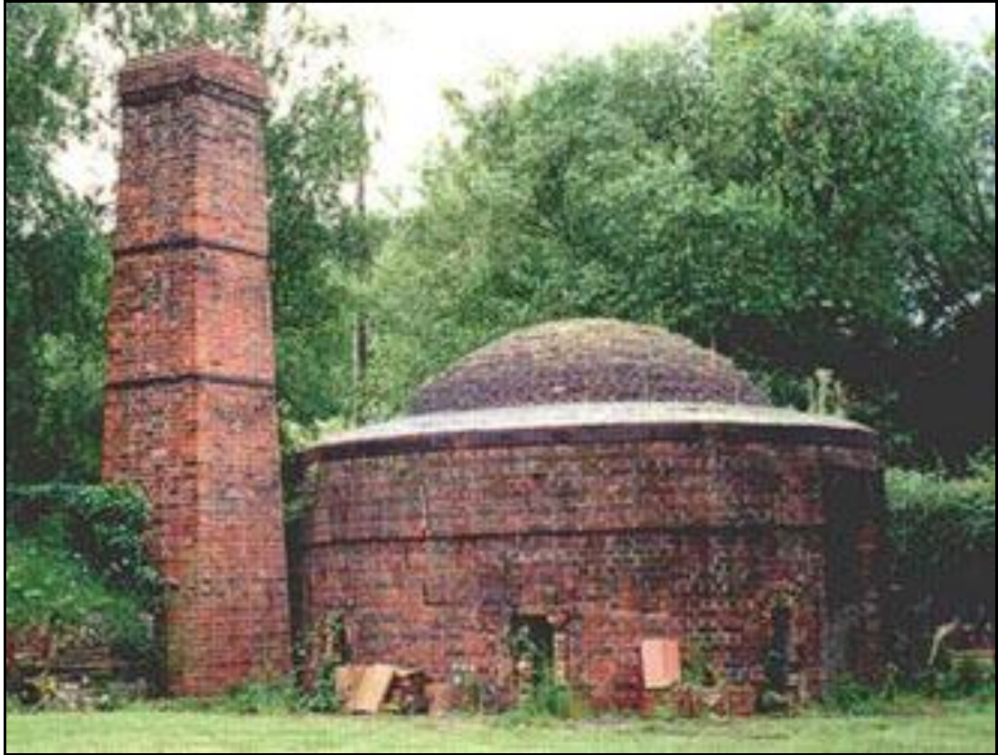
An illustration of a “Down Draft” kiln with adjacent chimney
