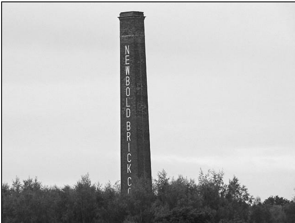
THE ICONIC "NEWBOLD BRICK COMPANY LTD" CHIMNEY BUILT AS A FLUE CHIMNEY FOR THE HOFFMANN 22 CHAMBER KILNS c.1933.
