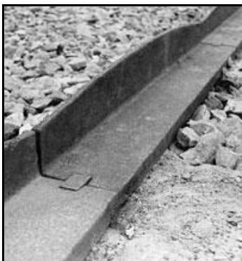
SECTION OF TYPICAL PLATEWAY RAIL
