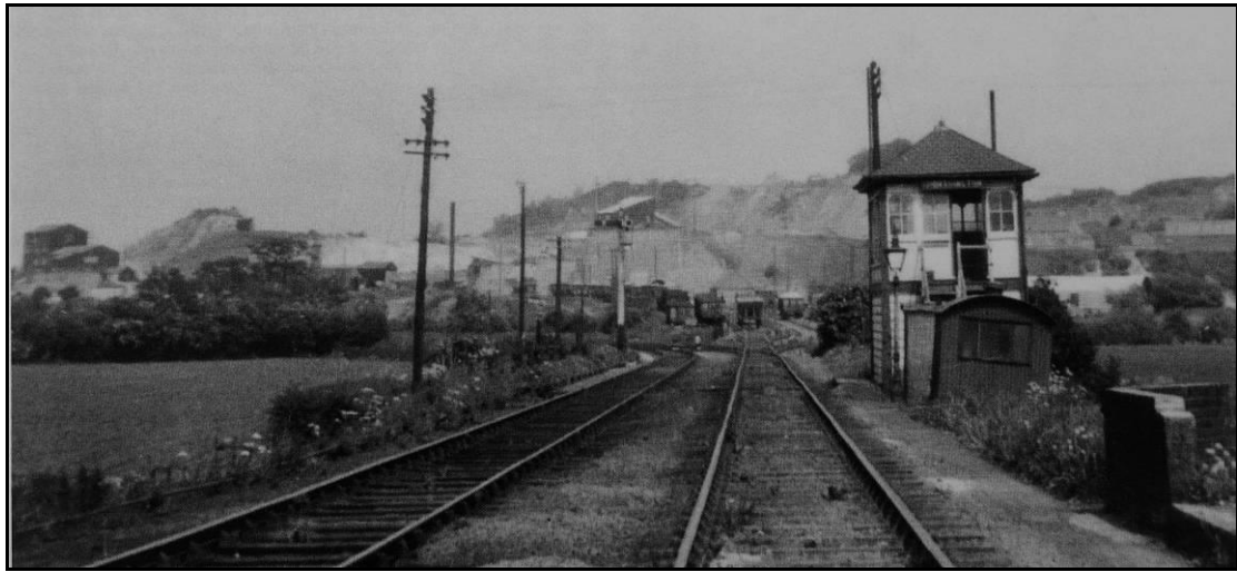
LOOKING DOWN THE RAILWAY TRACK FROM WORTHINGTON STATION VIA THE SIGNAL BOX TOWARDS CLOUD HILL QUARRY SIDINGS
