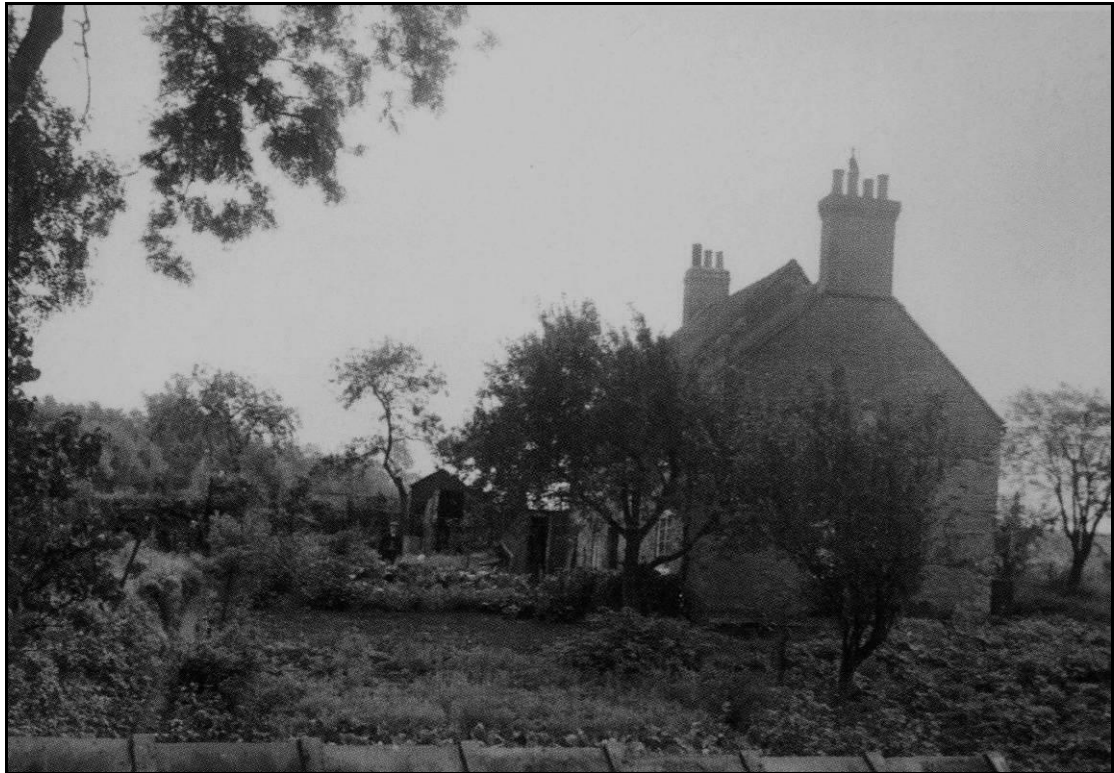
WOODSIDE COTTAGE c.1947 - DEMOLISHED IN 1965
