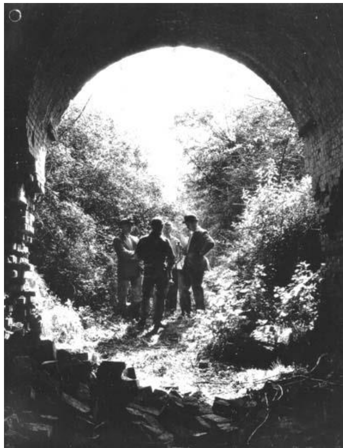
THE ENTRANCE TO THE CIRCULAR PEGGS GREEN BRICK TUNNEL AT ST. GEORGE'S HILL, SWANNINGTON WHICH HAS NOW BEEN FILLED IN
