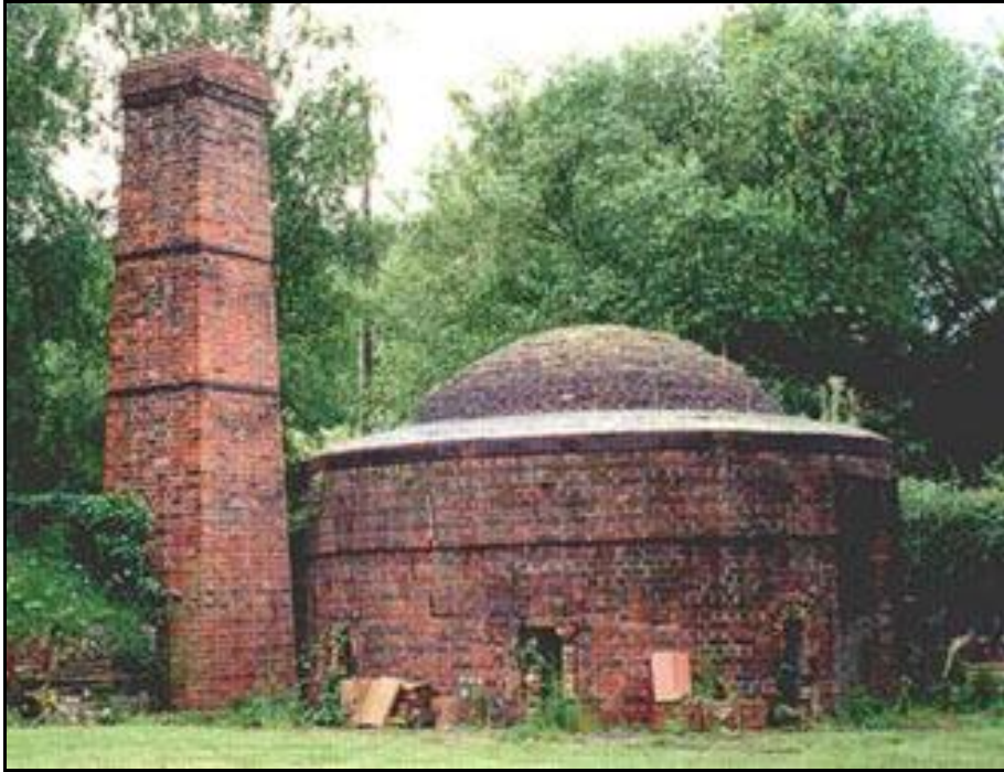
Intermittent burning down-draft type kiln
