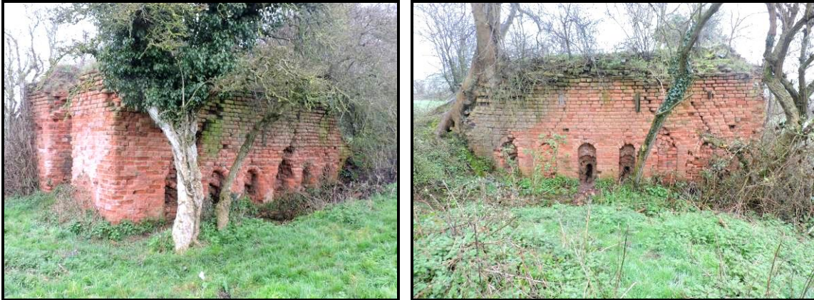
Remains of an up-draft “Scotch” kiln at Griffydam of the type thought to have also been used at Coleorton brickworks also
