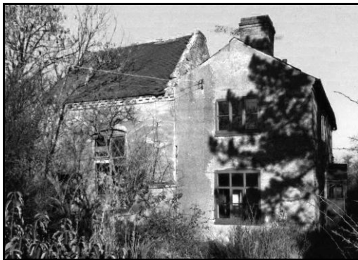
View from Gelsmoor Rd. with The remains of Chapel on the left
