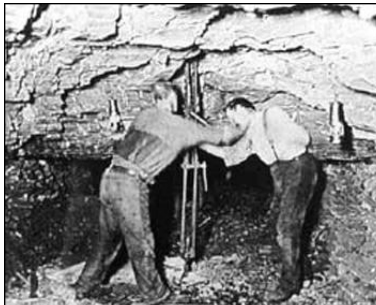
Example of hand drilling holes for explosive charges. Note the Davy safety lamps in the lower photograph
