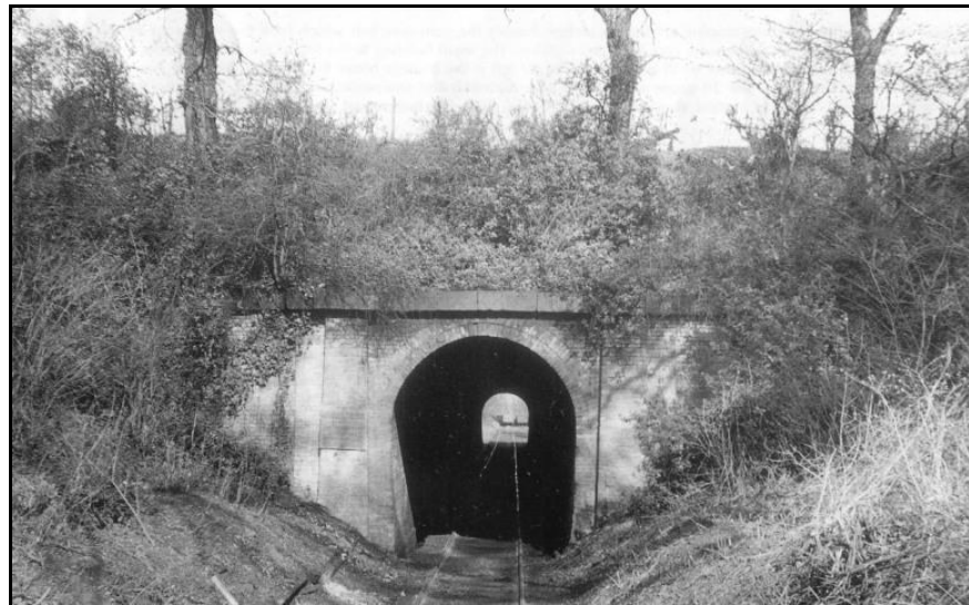
Before rails were removed
