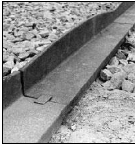
SECTION OF TYPICAL PLATEWAY RAIL
