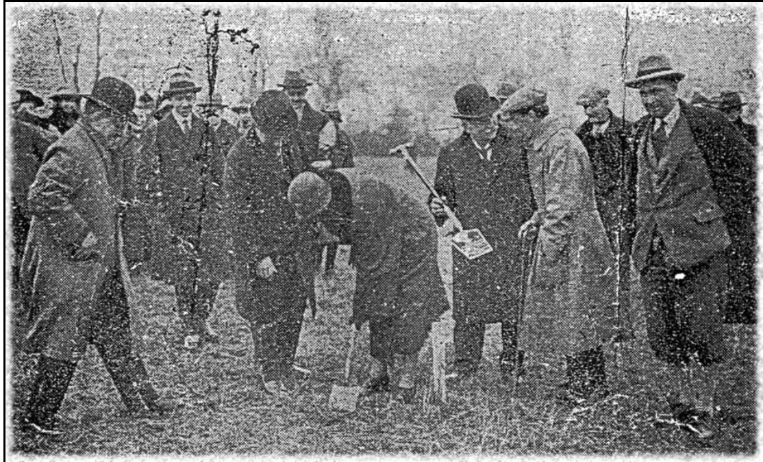
Lady Renee Beaumont turning the first sod on land at Newbold for the “New Lount Colliery” foundation on Friday the 8th of February 1924
