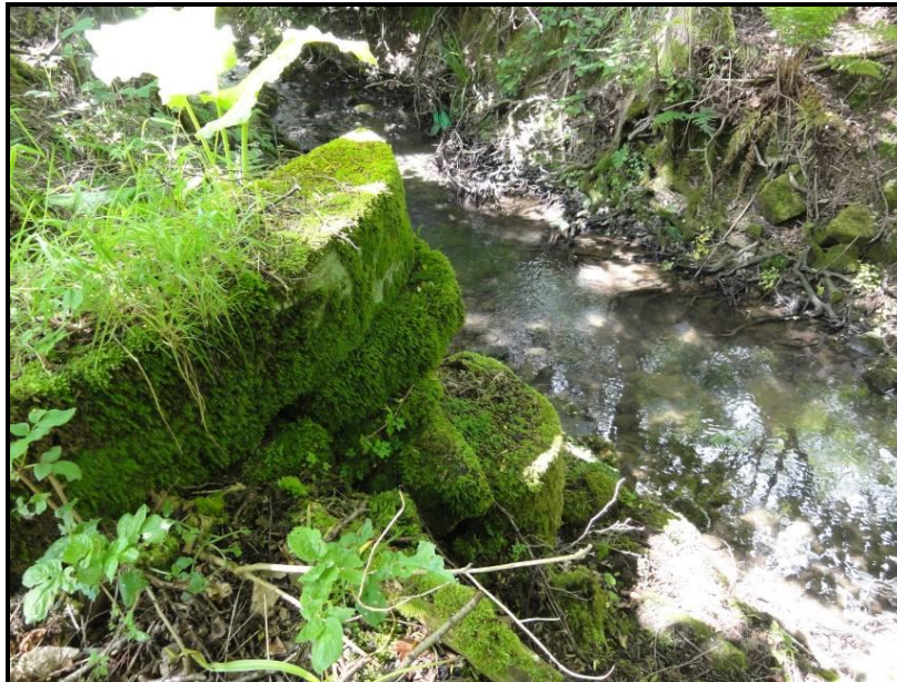
The above photograph shows the furnace or hammer pond sluice gate walls at the side of the brook, Note the accurately dressed radius on the ends of the stones.
