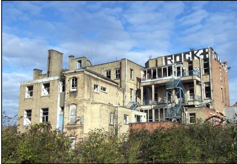
Loughborough General Hospital from the rear awaiting demolition
