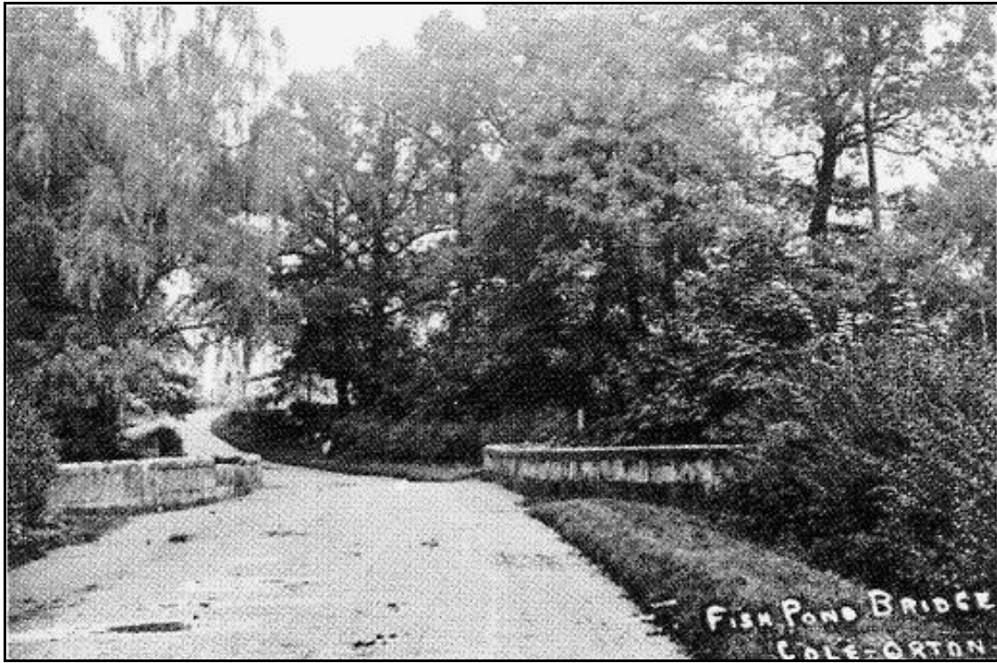
PHOTOGRAPH OF FISHPOND BRIDGE PRE 1938
