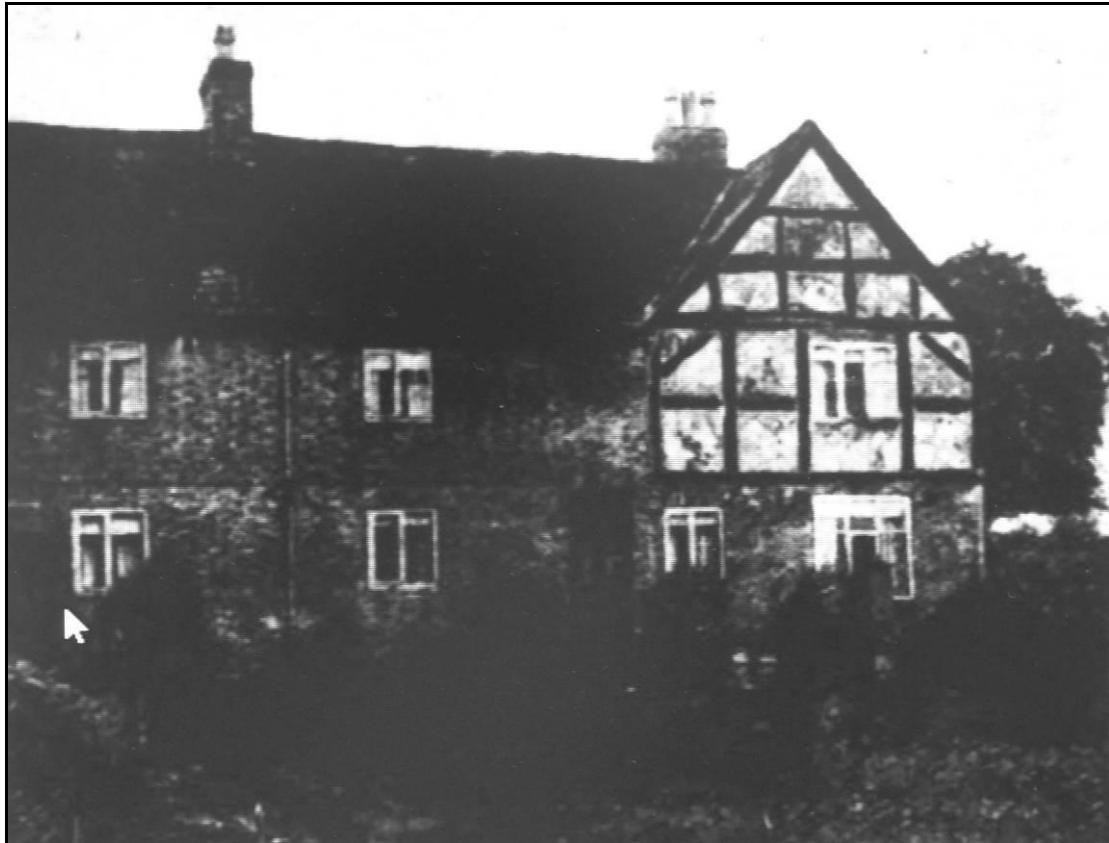
1939 photograph taken from side facing St. Mary's church
