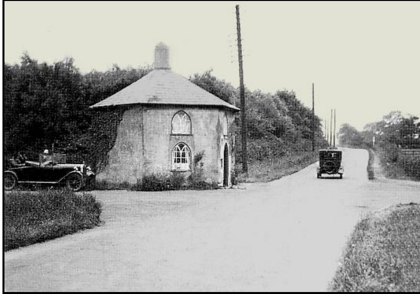
Lount Tollgate cottage c.1930. Taken from the Breedon side of the Breedon to Ashby Road. See the following Hansard report.
