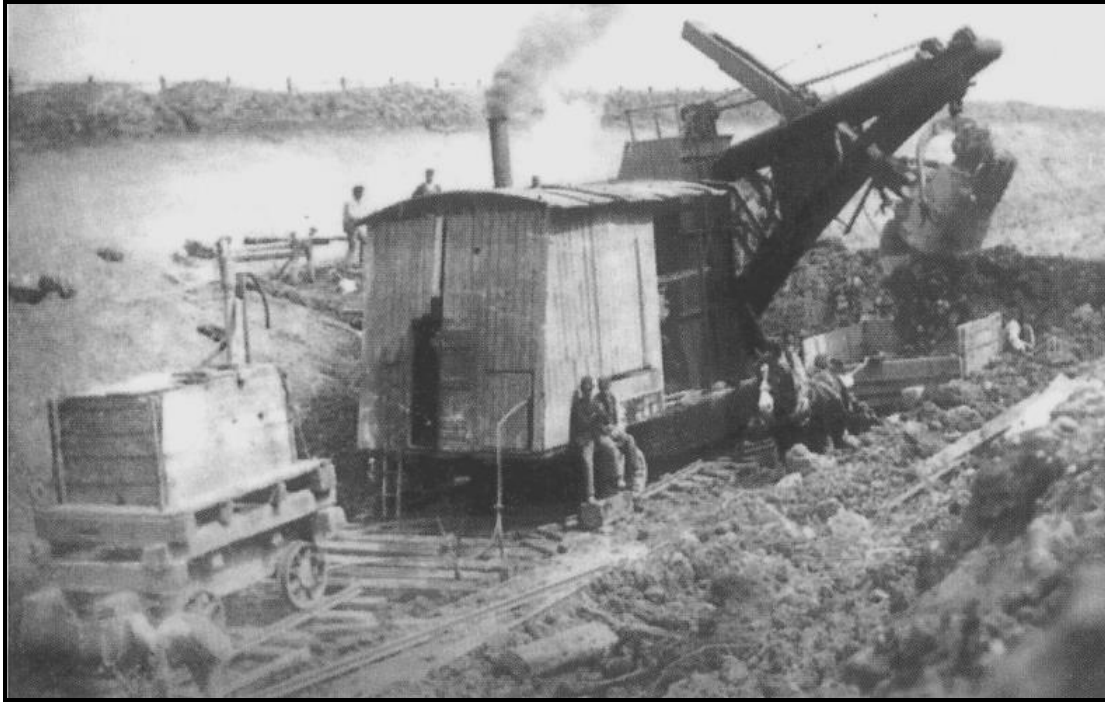
A Steam Navy working on the Worthington to Ashby section of the Derby to Ashby Midland Railway c.1872.
