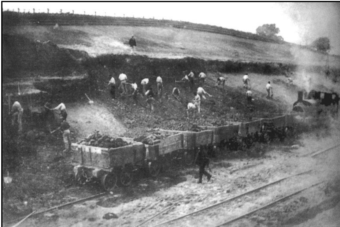
Digging a cutting on the Worthington to Ashby section of the Derby to Ashby Midland Railway c.1872. This section of the railway was opened on Jan 1 st 1874.
