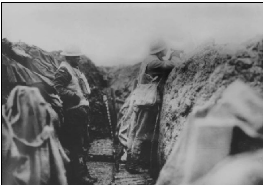
Biscuit Trench east of Flers, near Guedecourt,
