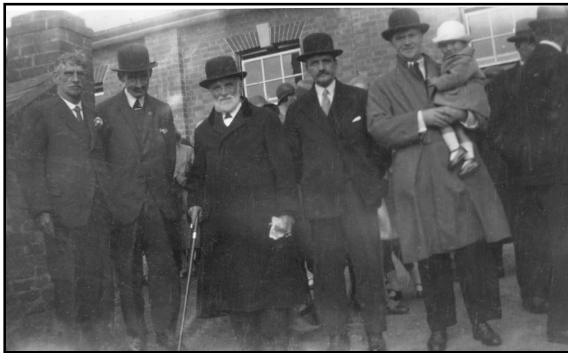
Photograph taken at the opening of the new Sunday School building in 1932 on the LH side of the Chapel. This was built by Ramsdens' of Castle Donnington
