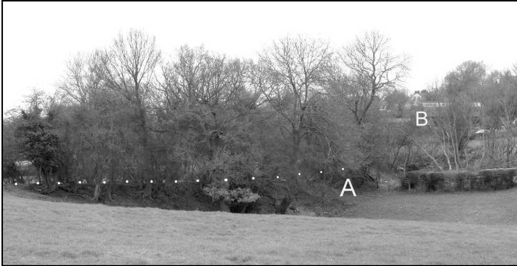
Photograph of the tramway embankment as it was in 2013. The tram rails have now gone of course, but the line of the embankment is highlighted by the white dots. A section in the middle had been taken out where marked A . The Griffydham Senior School building is in the distance marked B
