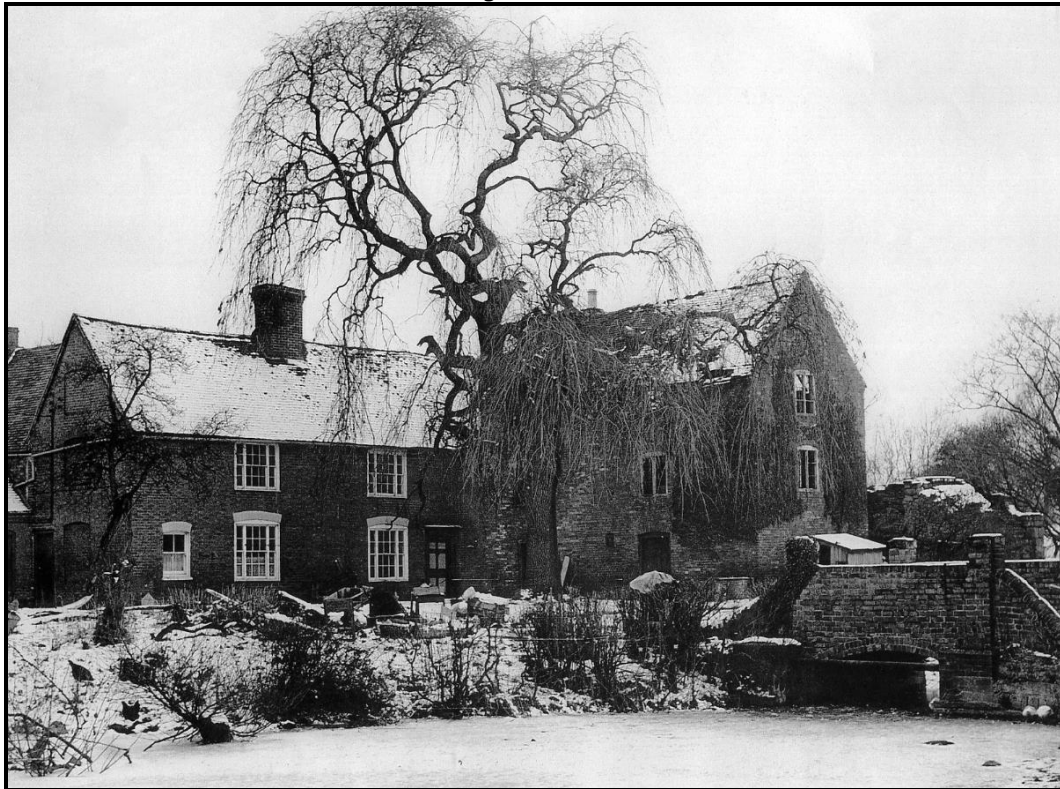
This photograph, although similar to the above, has the addition of a window on the left, and was taken later with snow on the ground. The building had clearly undergone some external refurbishment at this time, and there is evidence of the addition of a window.
