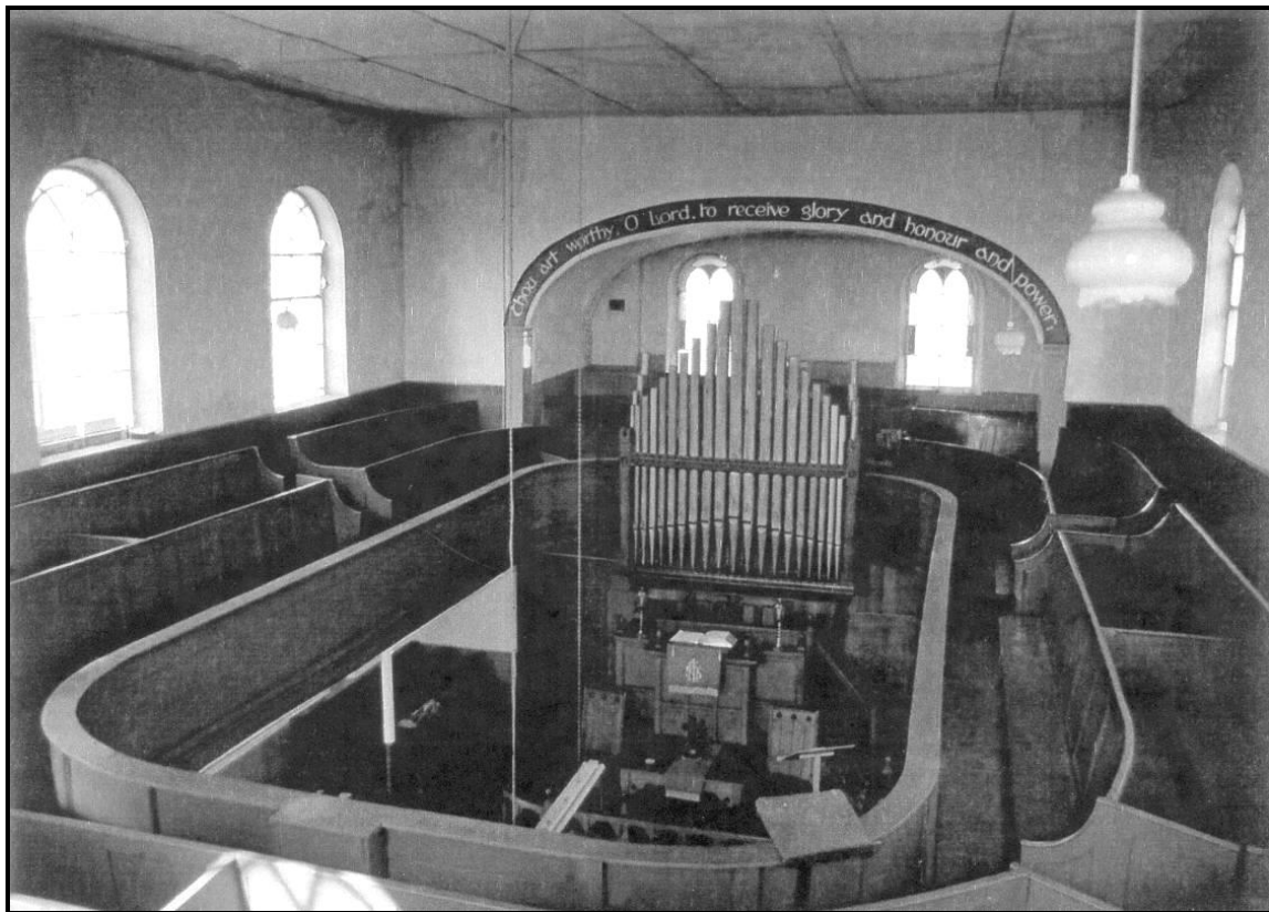
Internal photograph of Chapel taken from the upper gallery, thought to have been added during the chapel enlargement in 1862. The chapel then provided seating for approx 200 people.
