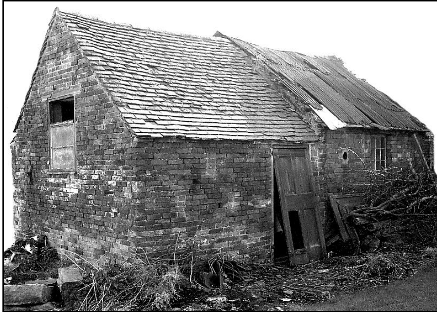
Charlie's nail shop and forge in the Woolrooms in 1988. This has now been preserved by the current owner of the property on which it stands
