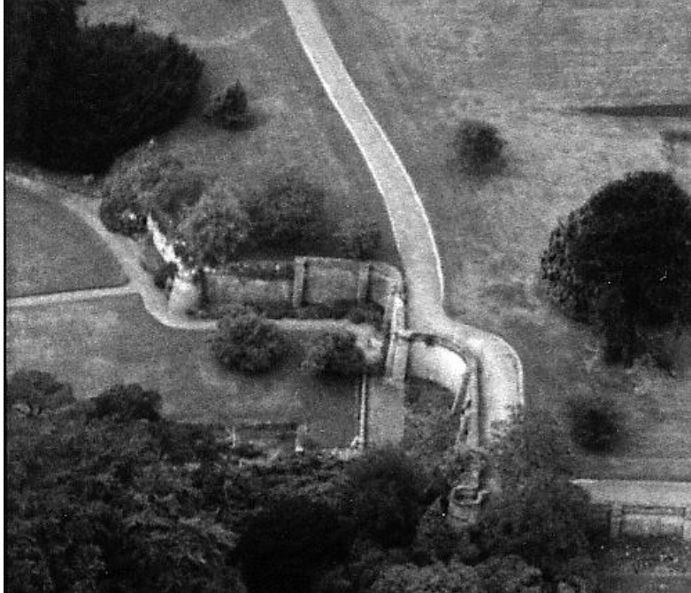
Aerial view of 4m high north retaining wall
