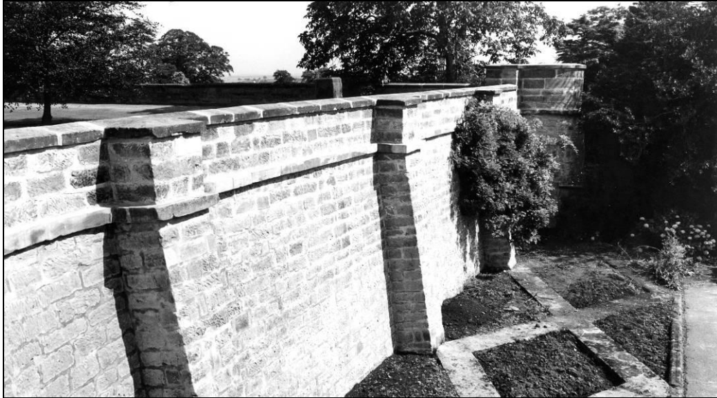
Eastern end of the 4m high retaining wall with a viewing “Pulpit” at the end. This is shown on Wordsworth’s plan at the north east corner. The photograph was taken after repairs to the wall were carried out in 1986.
