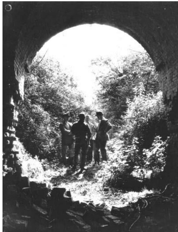
THE ENTRANCE TO THE CIRCULAR BRICK TUNNEL AT ST. GEORGE'S HILL, SWANNINGTON WHICH HAS NOW BEEN FILLED IN
