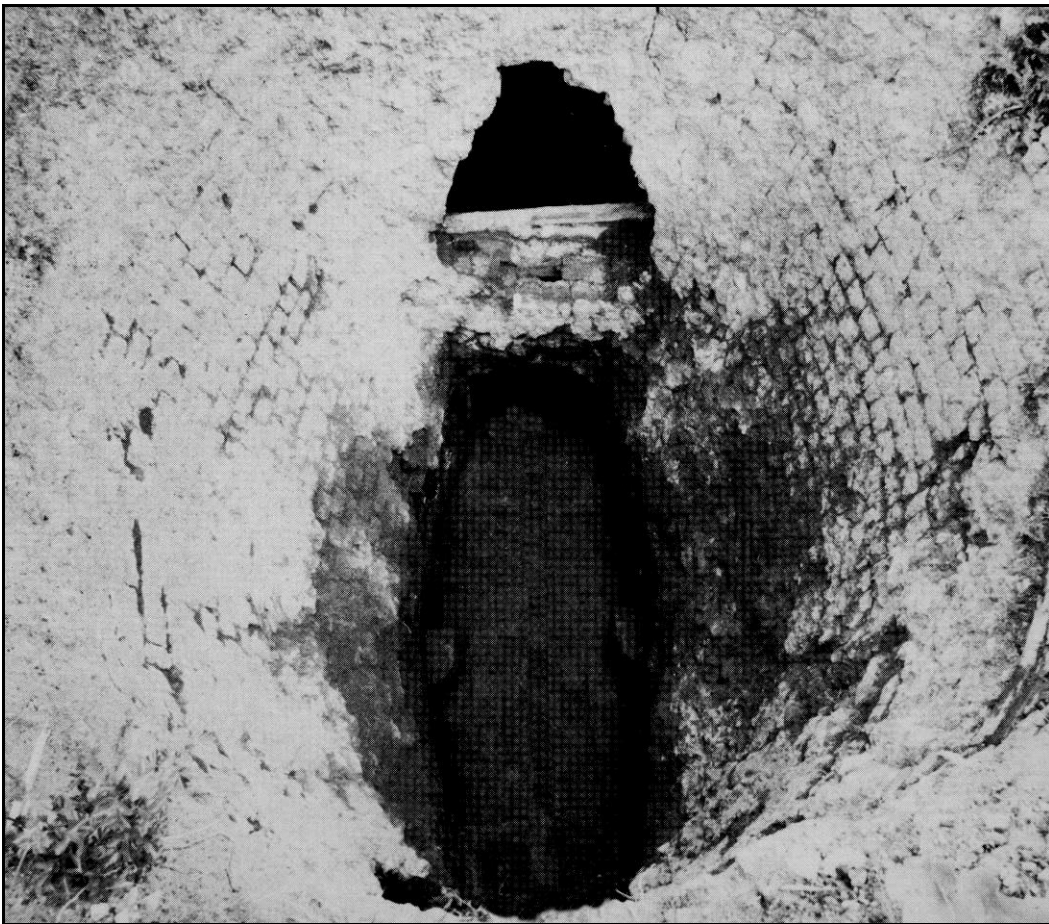
A MOIRA LIME KILN PHOTOGRAPHED PRIOR TO RESTORATION WORK
