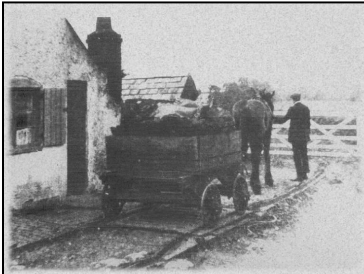
A Ticknall tramway wagon on the weigh-bridge between Old Parks Farm and Ashby. Note the removable wooden container mounted on top of the wagon chassis. Apparently, after the line closed in 1913, the Midland Railway Company made occasional trips over it to try and keep the "Right of Way" open, but it was officially closed in 1915.
