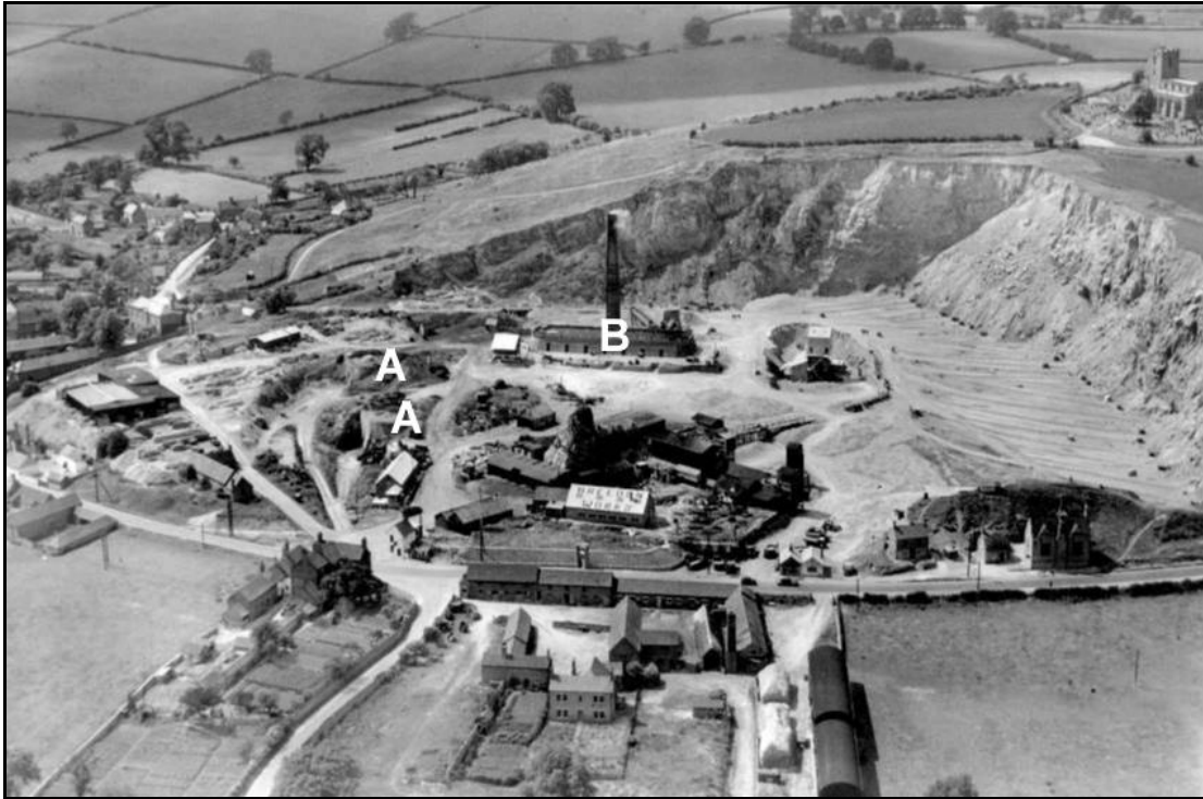
PHOTOGRAPH TAKEN IN 1936 JUST PRIOR TO THE 1937 BRITISH INDUSTRIES FAIR EXHIBITION. THE TWO LARGE ROUND LIME BURNING KILNS ARE MARKED A , BOTH OF WHICH HAD TO COOL DOWN BEFORE THE BURNT LIME COULD BE RAKED OUT AND LOADED INTO WAGGONS. THE SERCOMBE CONTINUOUS BURNING MULTI-CHAMBER KILN IS MARKED B . THIS WAS IN OPERATION AT THIS TIME AS THE CHIMNEY CAN BE SEEN SMOKING
