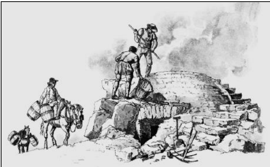
A LIME BURNING FIELD FLARE KILN - 1806 AN ETCHING BY W H PYNE
