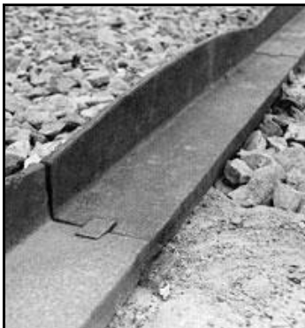
SECTION OF TYPICAL PLATEWAY RAIL
