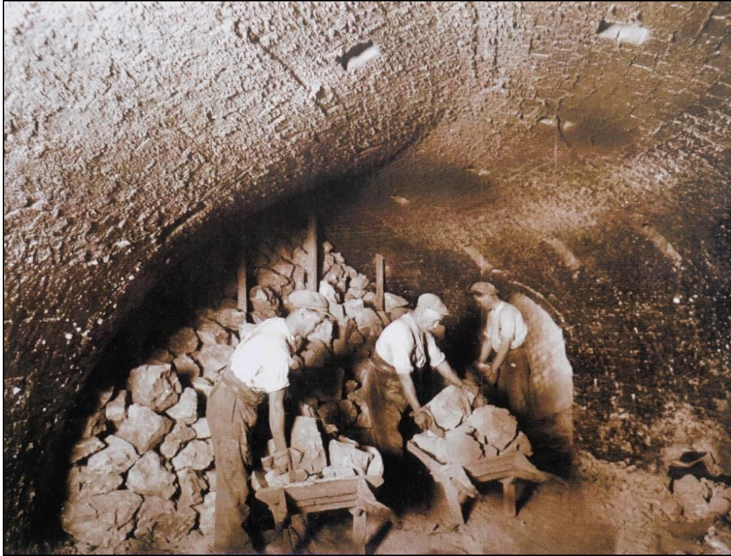
RECHARGING THE SERCOMBE KILN AT CLOUD HILL WITH LIMESTONE
