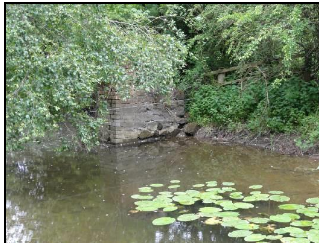
The broken out brick arched culvert a few yards from the edge of the lake as described above
