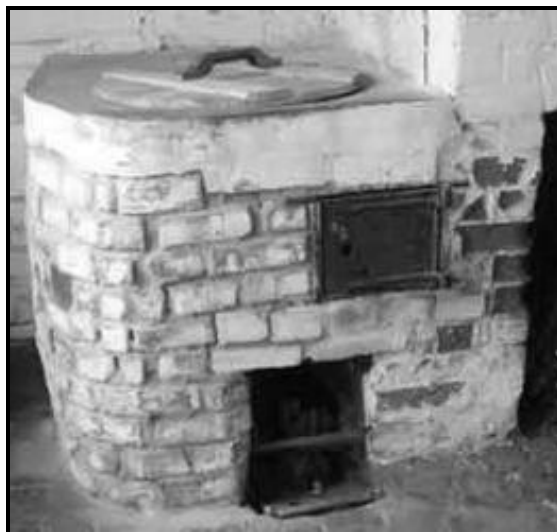
A small copper boiler with the copper cauldron covered with a wooden lid for safety - the fire box is at the bottom
