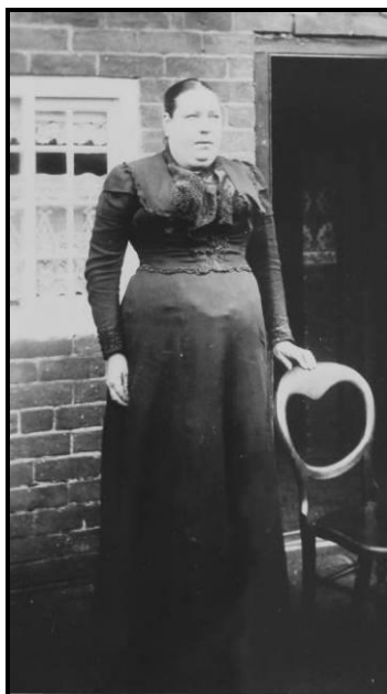
Mrs. Eyre outside Laundry House (This is the RH door at the end of Laundry House in the above photograph)
