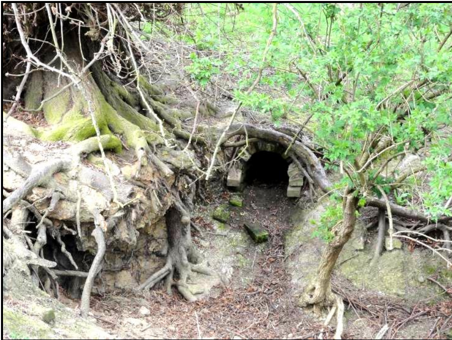
The broken out brick arched culvert a few yards from the edge of the lake as described above
