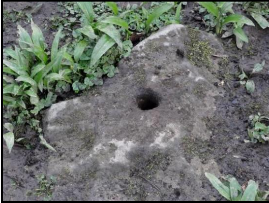
The two sleeper blocks found on top of the bridge In some cases, it was necessary to dress the sleeper blocks to provide a flatter surface for the rails to sit on, as shown in the RH photograph.
