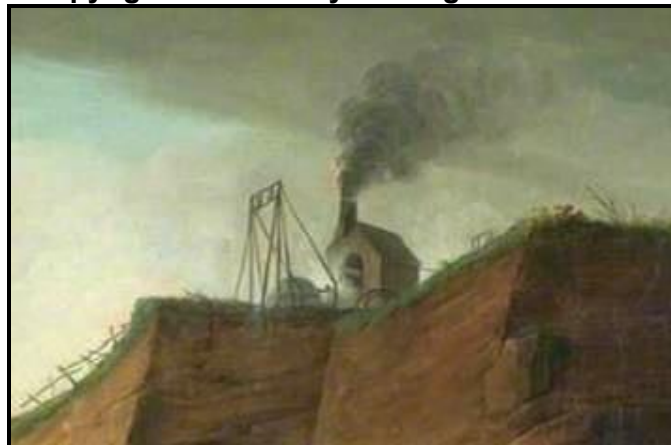
Enlarged view of winding engine house on the top rim of the quarry, which also depicts a semi-circular haystack boiler (see following text).
