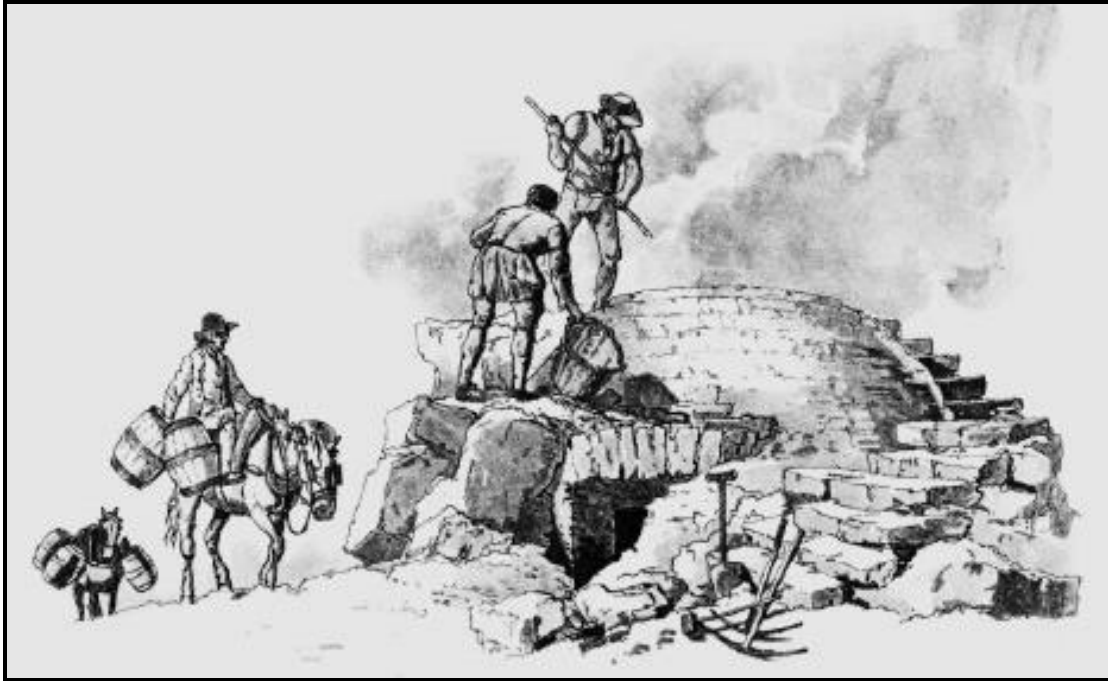
An etching from W. H. Pyne 1806 of a typical Field Lime Kiln with fuel being brought by packhorse. It is not difficult to visualise that this may have been typical of the first kilns built by Earl Ferrers, which bears some relation to the mystery stone arch.
