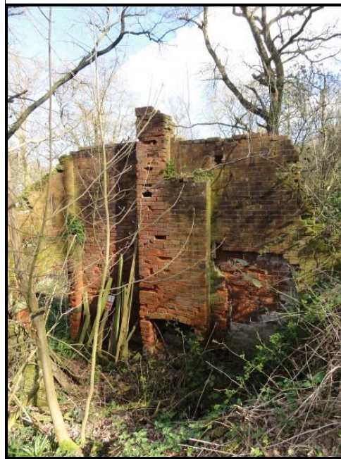
Photographs of what remains of the office. This was clearly part of a larger building and foundations confirm this. It is almost certain that this incorporated the chimney to which the flue came from the cupola furnace as described above.
