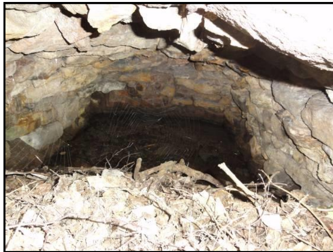
The above photograph shows what can be seen of the inside of the archway where the lime was raked out.
