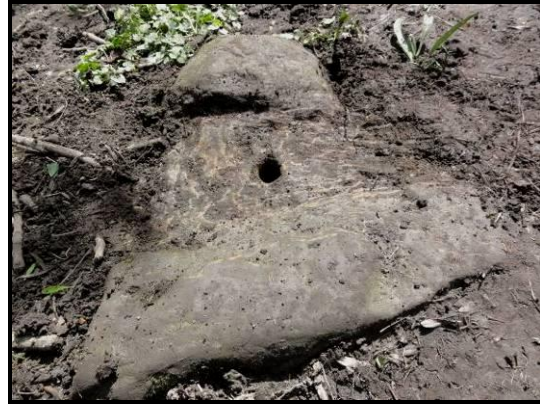
The two sleeper blocks found on top of the bridge In some cases, it was necessary to dress the sleeper blocks to provide a flatter surface for the rails to sit on, as shown in the RH photograph.
