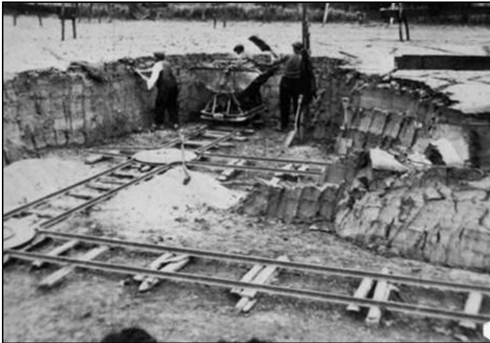
A typical clay pit. Note the turntables and tramway which would have led to the brick making area
