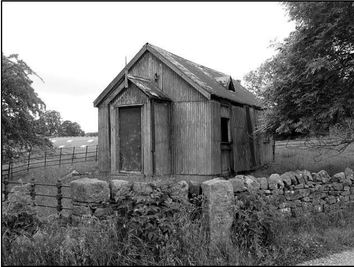
A TYPICAL ABANDONED METHODIST TIN TABERNACLE IN YORKSHIRE SIMILAR TO THE ONE USED AT LOUNT FOR THE PRIMITIVE METHODIST CHAPEL (SEE INSIDE PAGE)
