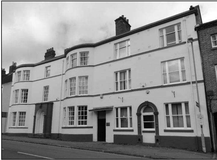
Front view of Fisher's Solicitors offices 2014
