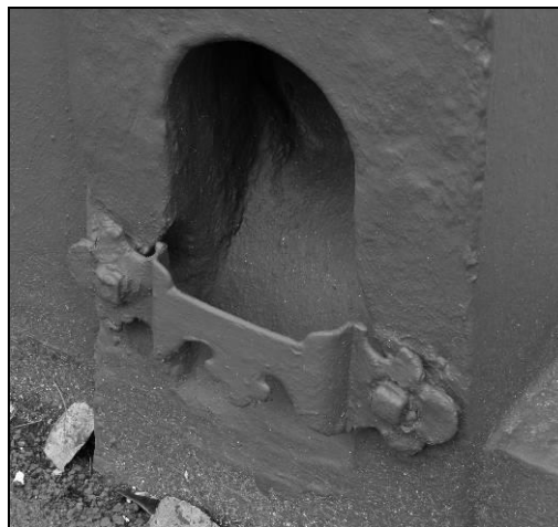
Close up of boot / shoe scraper on front of former R.H. doorway.
