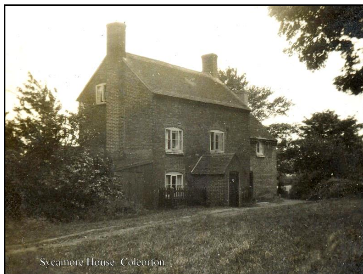
Sycamore House in 1936 when viewed from the front
