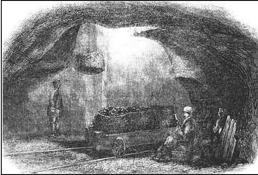
Illustration of corves (baskets of coal) being winched up the mine shaft. Note - the corves are now being transported in a tram on rails instead of on a sled
