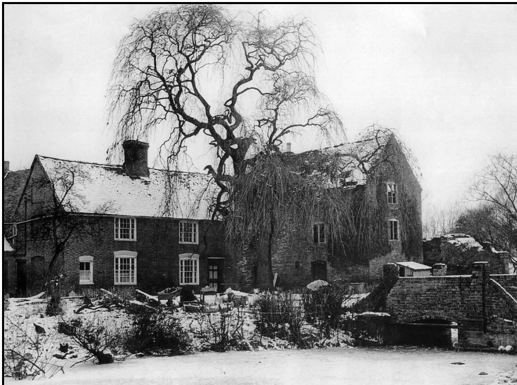
This photograph, although similar to the preceding one, has the addition of a window on the left, and was taken later with snow on the ground. The building had clearly undergone some external refurbishment at this time, and there is evidence of the addition of a window.
