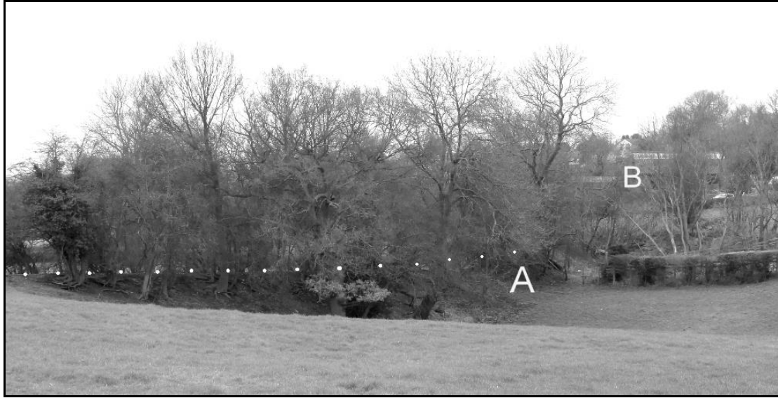
Photograph of the tramway embankment as it was in 2013. The tram rails have now gone of course, but the line of the embankment is highlighted by the white dots. A section in the middle had been taken out for access by the farmer where marked A . The Griffydam Senior School building is in the distance marked B . Photograph taken from Clay Lane end.
