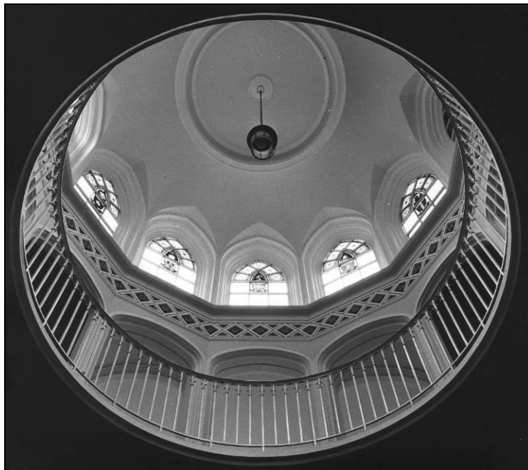
The polygonal Hall gallery and ceiling c.1960
