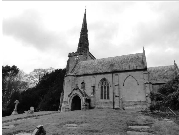
Northern (top) and southern elevations of St. Mary's Church in 2015.
