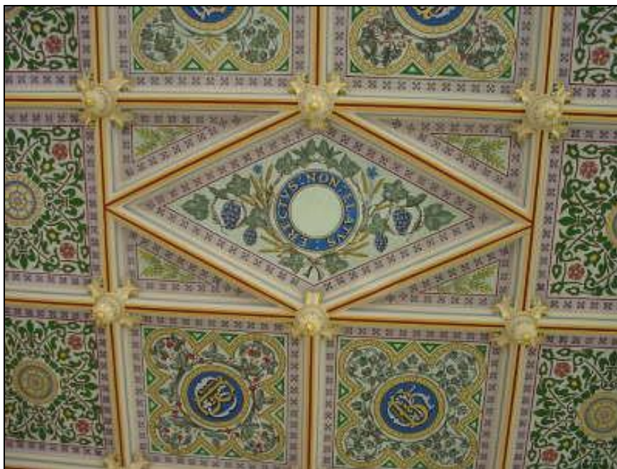
The re-painted ceiling in the Dining Room (Beaumont Room)
