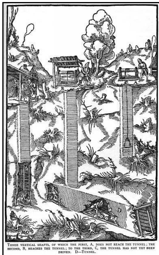
Timber lined shaft mining showing underground wagons running on rails
