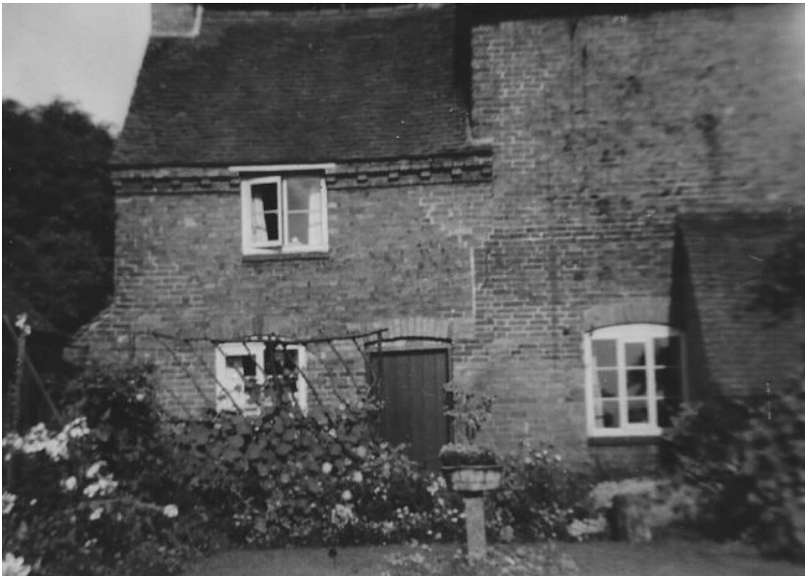
Part of the cottage pre-1960s
