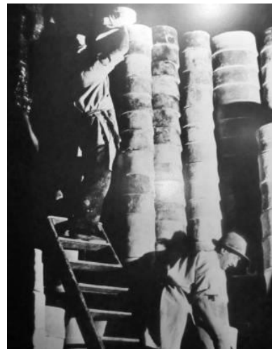
Loading Saggars into a kiln
