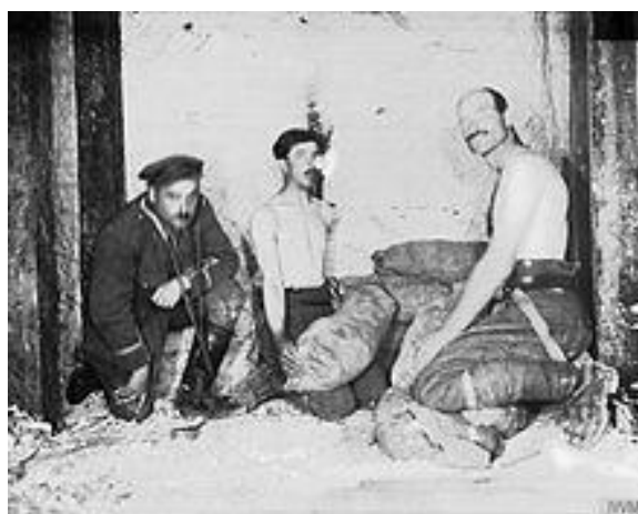
Miners laying charges for one of the mines on the Somme, 1–13 July 1916.
