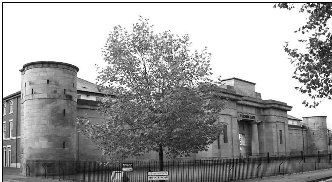
The retained facade of Vernon Street Gaol
