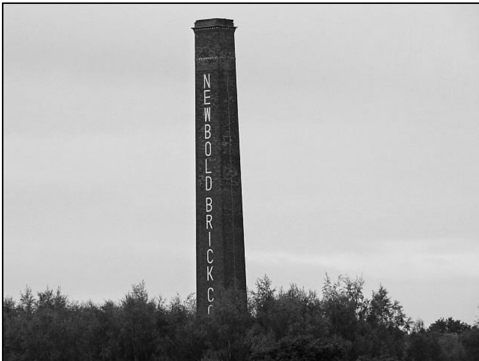
Newbold Brick Co Ltd chimney
