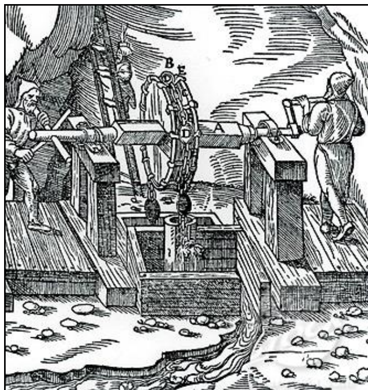
A ‘Rag and Chain Pump’ used to pump water from the pit bottom.
