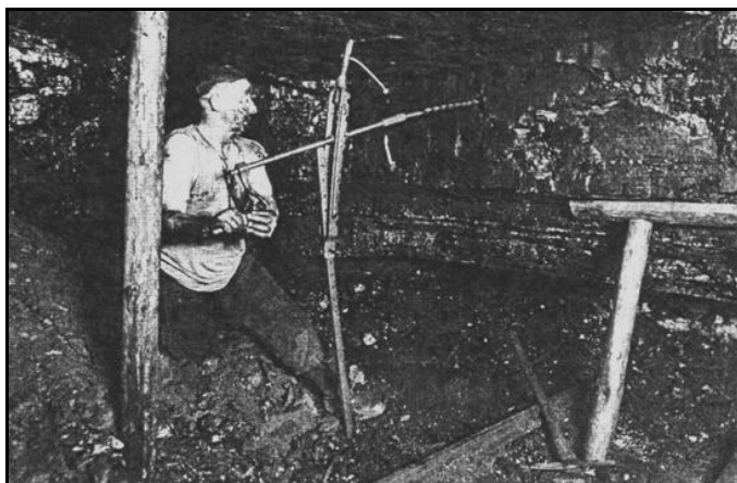
Hand drilling holes for explosives (photographs from the healeyhero website, thought to be of Staunton Colliery)
