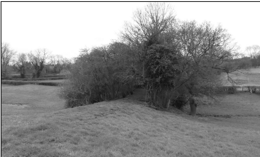
View on end of the embankment from Clay Lane, Peggs Green direction in 2013
