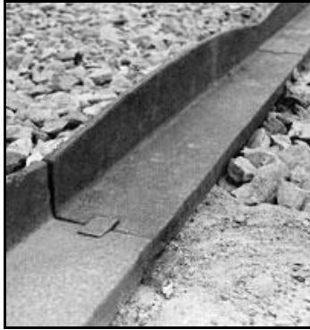
Section of typical Plateway rail
