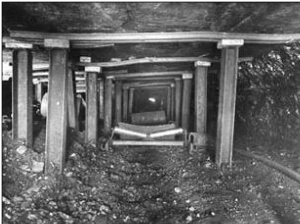
Photographs of typical “Long Wall” working in the early 20th th century where iron girders had replaced the previously used wooden pit props, and conveyors were starting to be installed. The first conveyor was installed in Yorkshire in 1902.
