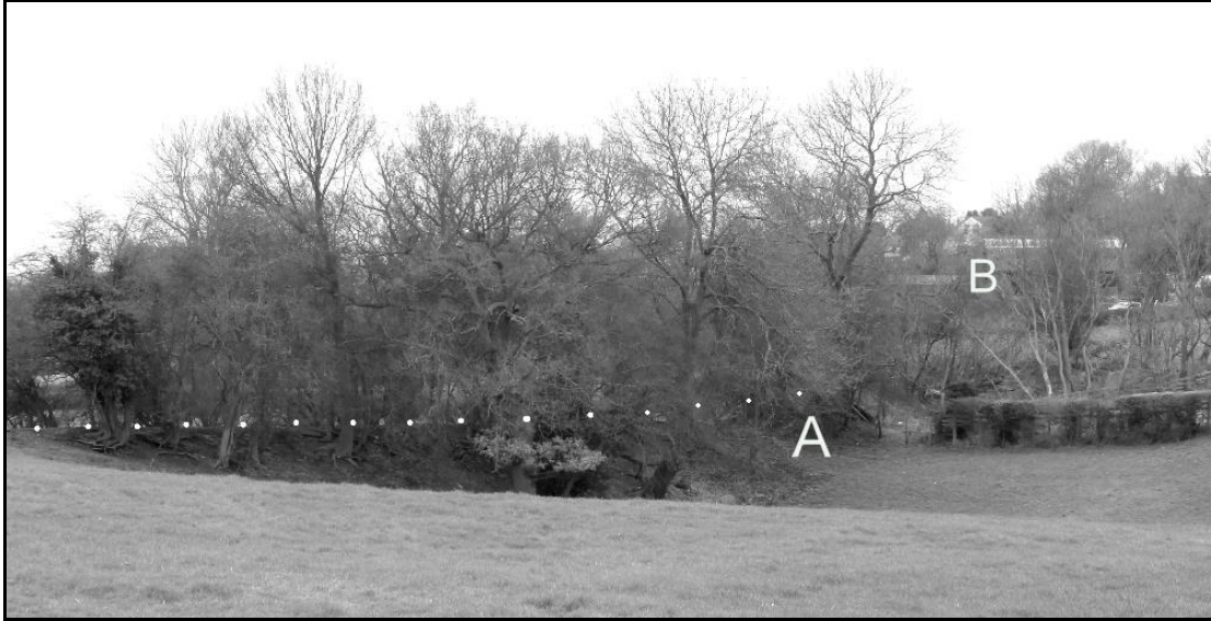
Photograph of the embankment as it is in 2013. The tram rails have now gone, but the line of the embankment is highlighted by the white dots. A section in the middle has been taken out where marked A. The Griffydam Senior School building is in the distance marked B
