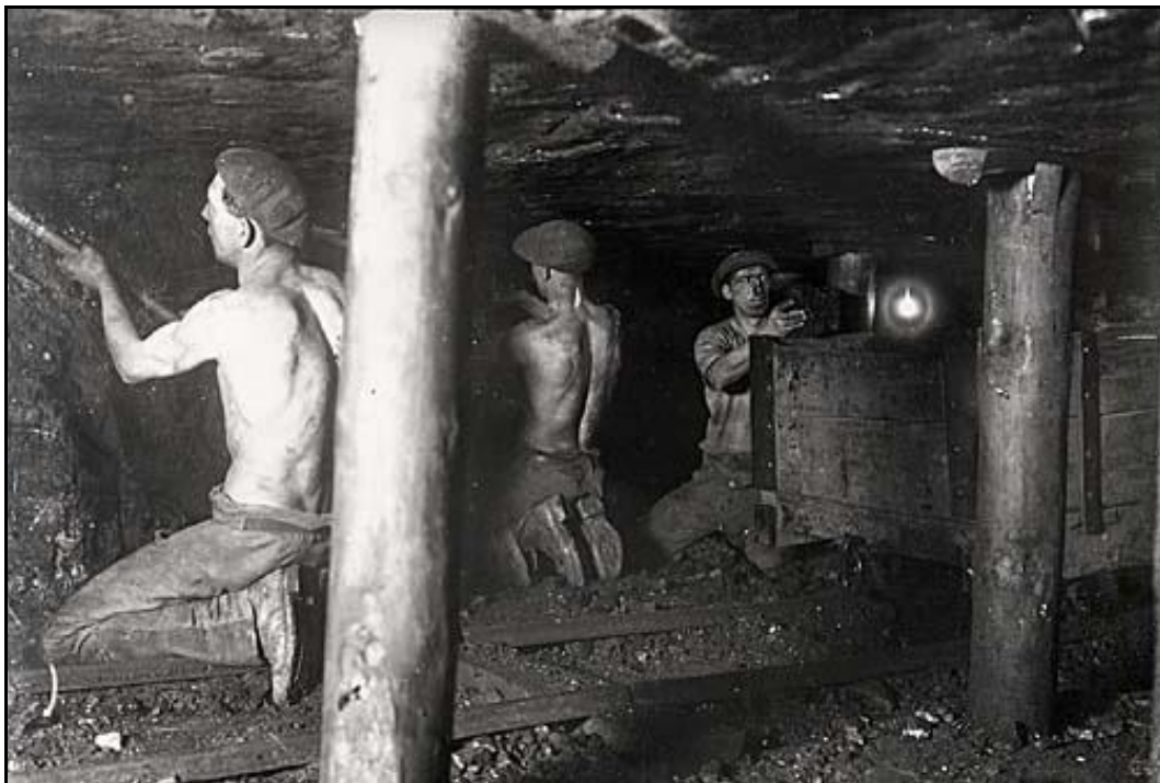
Miners working a "Long Wall" face
