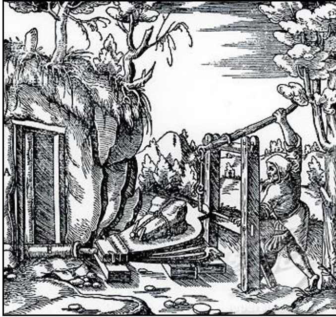
Ventilating a mine using bellows
