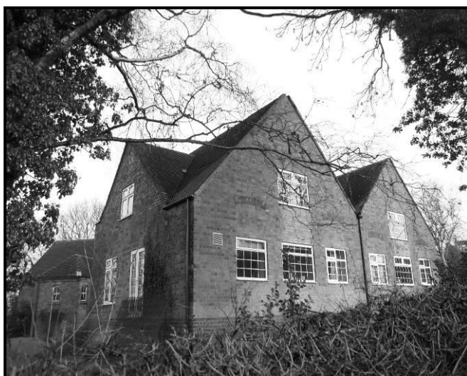
Photographs of Griffydam Senior School taken just prior to it being converted into a private residence
