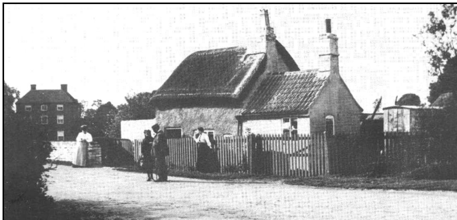
Early 20 th century photograph of single storey thatched cottage on Dawson's Rd (formerly Pol Matchet's Lane). The walls of the original part of this cottage in the centre were made from "Wattle and Daub" and possibly dates the original building back to the 1500's.
