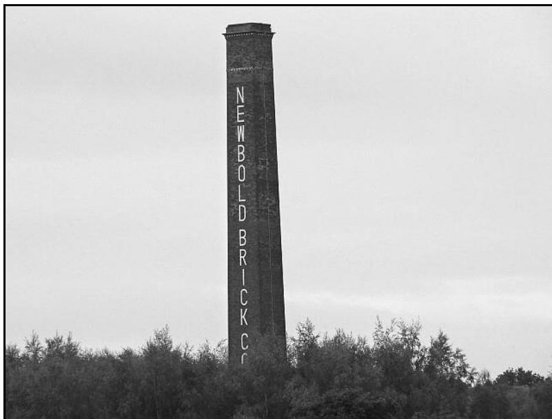
Newbold Brick Co Ltd chimney
