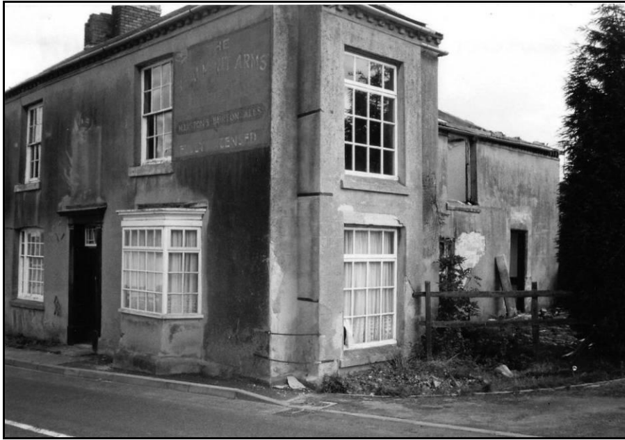
The Beaumont Arms building in 1994
