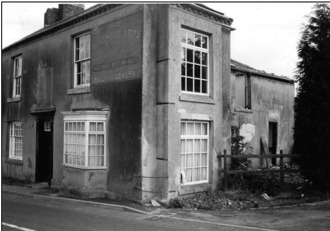
The Beaumont Arms in a state of disrepair 1994
